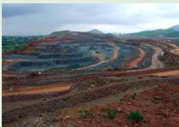
It is the first opencast uranium mine of the country and was commissioned in January 2009 with a capacity to produce 3500 tpd ore. Situated adjacent to Turamdih Mill, the deposit contains a moderately large reserve with very low uranium content. It is a conventional opencast mine using excavator-dumper combination. It has ore benches of 6m height, over burden/waste benches of 6m/12m height. The pit will attain
