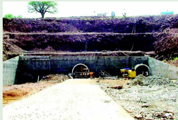
Construction of an underground mine and plant with a capacity of 3000 tpd near Pulivendula in Kadapa district of Andhra Pradesh is progressing satisfactorily. The mine entry is being constructed with three declines with ore planned to be hoisted through a conveyor. The plant shall have alkali leaching process under pressure. The project is expected to be commissioned during the year 2011.
