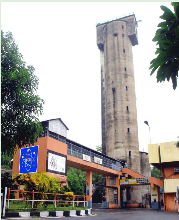
650 m depth. Various modifications and standardisation with regard to roof support, stoping methods, machinery utilisation, stowing etc. have been carried out for optimum recovery of ore. Jaduguda is the deepest operating underground mine of the country with inherent deep-mining concerns like ventilation, strata control, rock temperature etc. The capacity utilization of the mine during the year was 55.9% compared to 61.31% during previous year.
